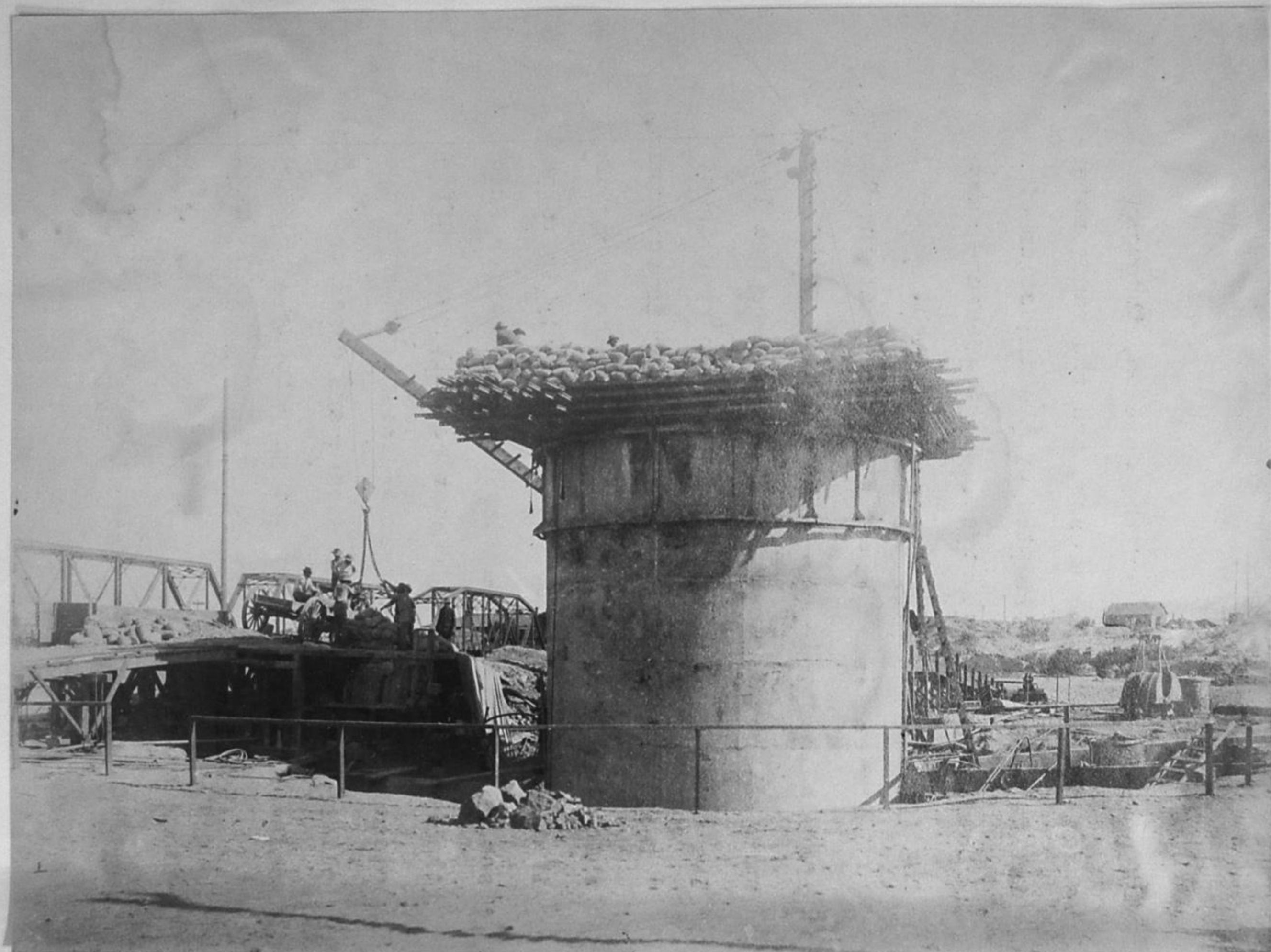
Fig. 18. California Caisson - 300 Tons Additional Load.
